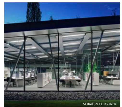
The slanted supports eliminate further bracings.
